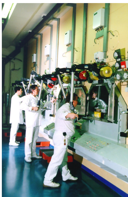
Photo n°2 : C10 Hot cell – General view
