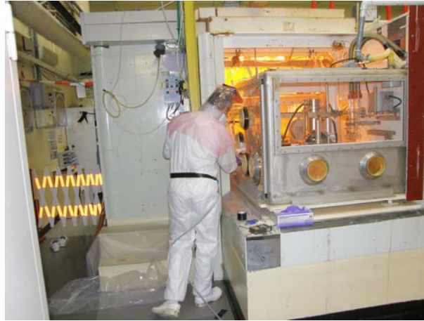
FIG. 3.1. Dismantling the old hot-cell.
