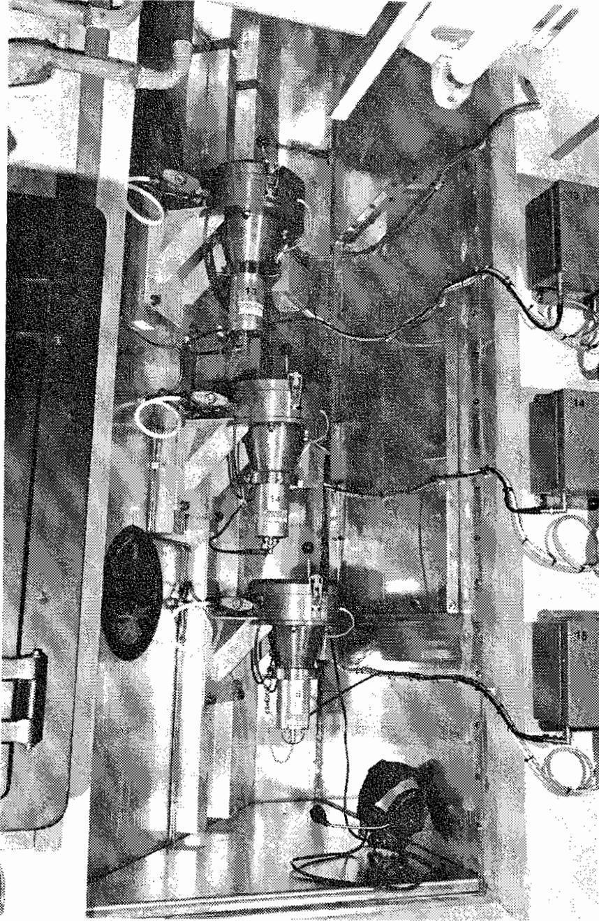
Fig. 3.3. Arrangement of the 2-of-3 system in the ventilation channel.
