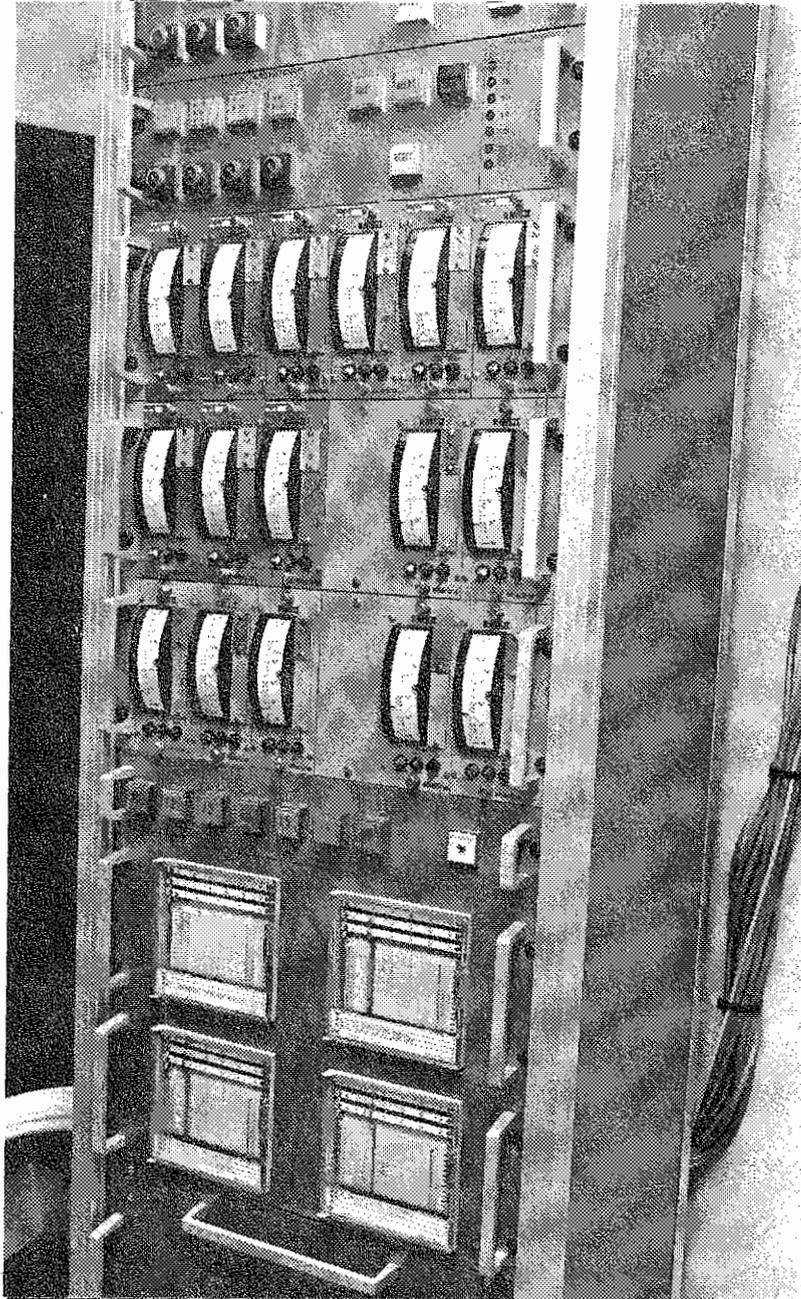
Fig. 3.6. Control board rack with rate meters, recorders, signal lamps and activation switches.
