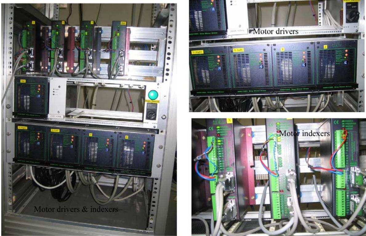
Fig. 4. Motor drivers installed in a rack outside the concrete cell.
