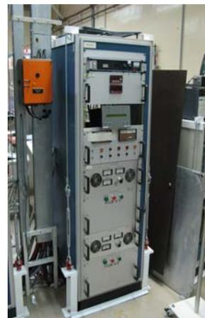
Fig 2 : Anchoring an electrical cabinet that represents a potential missile threat to a glove box
