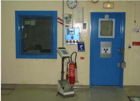
Fig 3 : Cell doors and glass panels were replaced with fire doors and panels to prevent any loss of leaktightness
