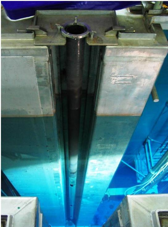
FIG. 3.3. Shows the inspection bay for the CC in the SFP.
