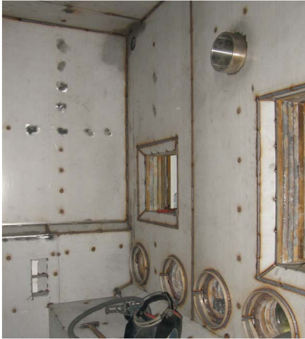
FIG. 2.1. Welding of inner stainless steel layer.
