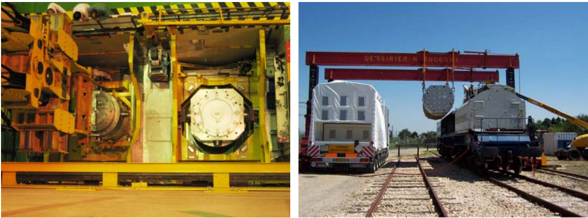
FIG. 6.2. ISAI is equipped to handle very heavy casks such as the TN 17.2 (at right on the picture on the left), which can be then shipped by railway (picture on the right).
