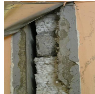
Opening of a joint in LEFCA: polystyrene and concrete
