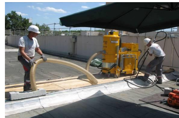
Removal operation from the roof
