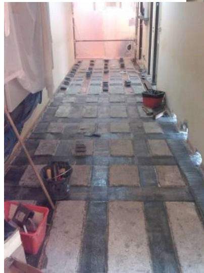
Reinforcement on the surface and underside of a floor.
