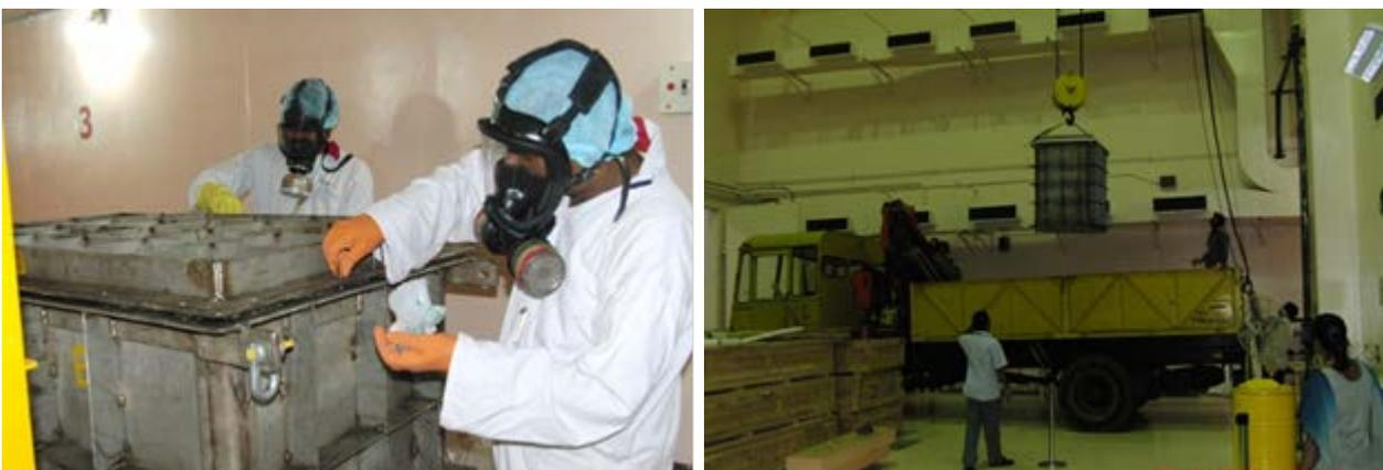
Fig 5 Disposal of CNC machine in leak tight containers and its transport.
