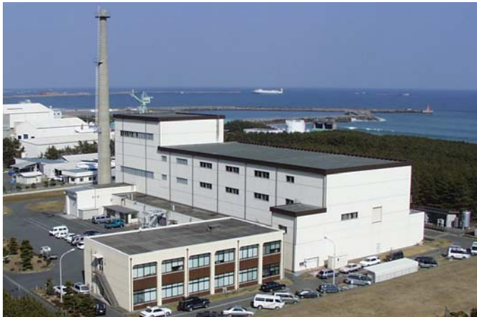
A view of the facility
