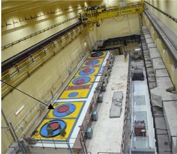
Figure 2: Hot cell roof with rotating roof plug assemblies.
