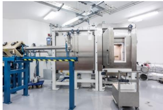
Newly installed hot cell
