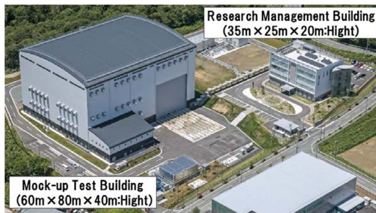
Fig. 1 Bird's view of the Naraha Remote Technology Development Center located in the Naraha south industrial park. The photo was taken in June 2016. The total area is 36000 m 2 .
