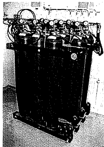
The new Inergen tubes, 1998.
