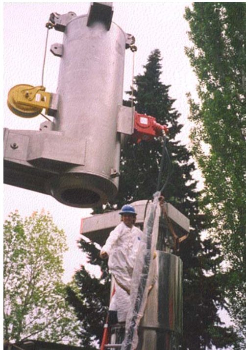
Figure III – Dry Transfer System (DTS Cask and Adapter)
