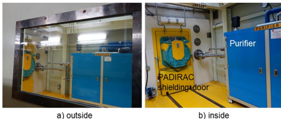
Fig 5. A refurbished isolation room of ACPF
