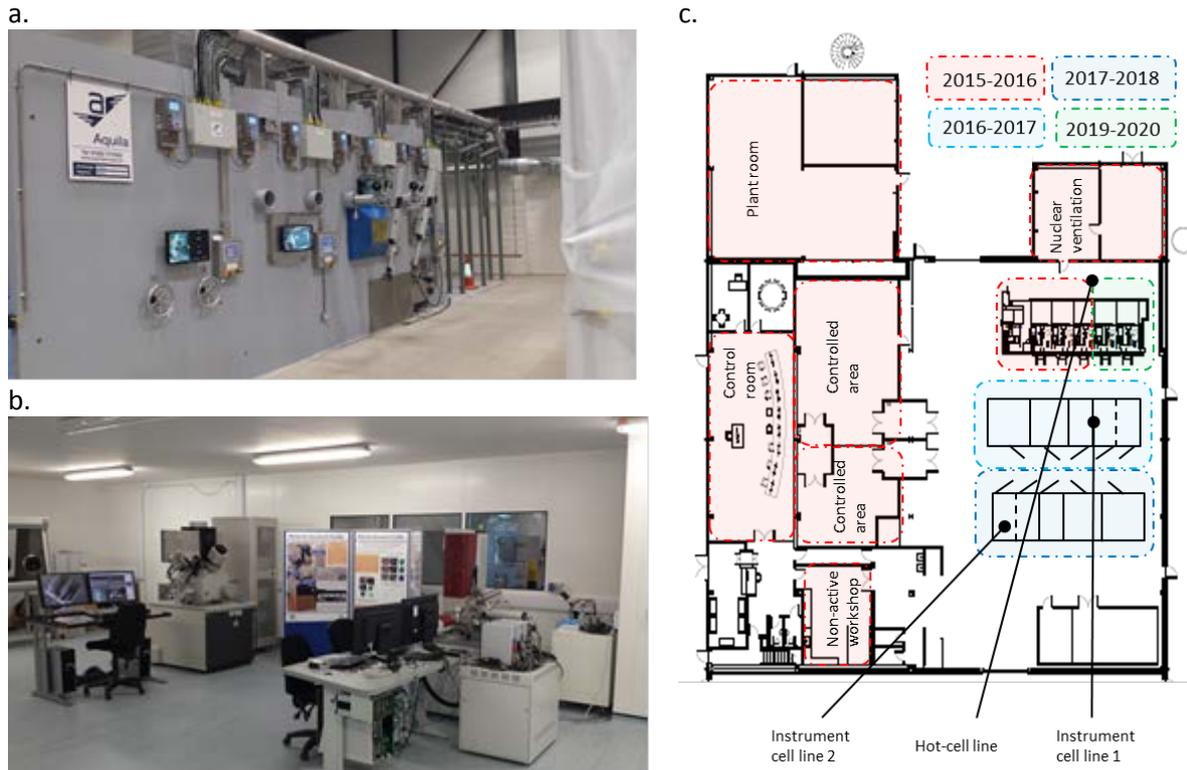
**Figure 2 UKAEA MRF facility with a. the hot-cell line; b. the FIB and SEM in the controlled area; c. Layout and current status of development**
