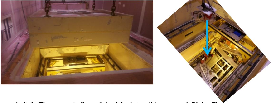
**Figure 4 : Left: The concrete floor slab of the hot cell is removed. Right: The measurement system is introduced inside the hot cell.**
