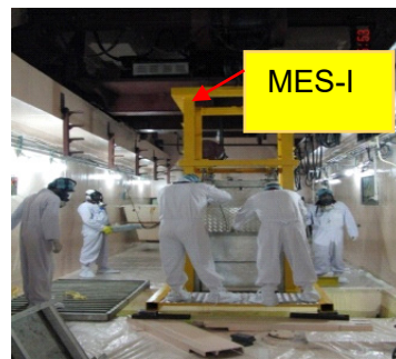
Fig.8 Man Entry System - I
