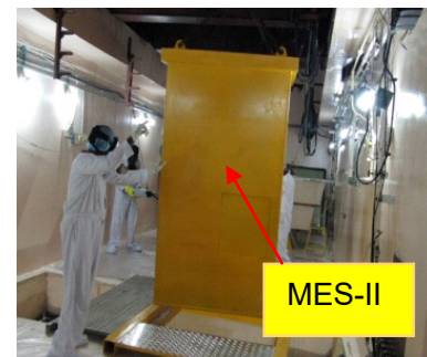
Fig.9 Man Entry System-II
