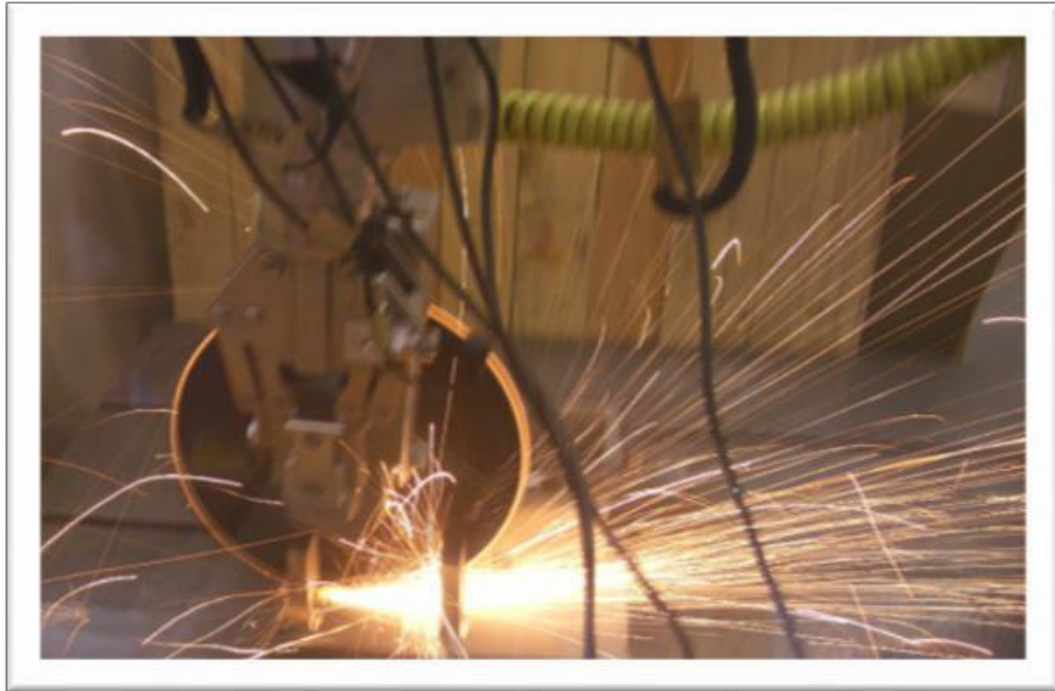
Fig. 4. Cutting with angle grinder
