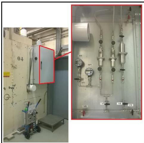
Figure P37: Valves system for gas sampling
