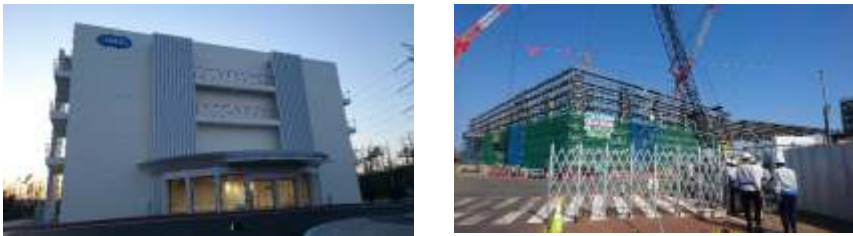
Figure 2. Administrative building (left), Laboratory-1 (under constructing) (right)
