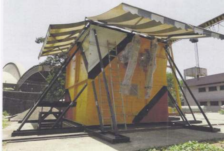
Figure 1: Mobile Hot Cell Installed at BRIT Vashi, Navi Mumbai, India
