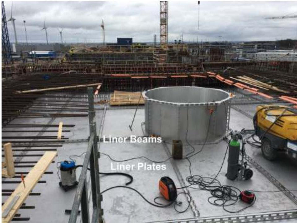
**Figure 2** Ceiling liner beam and plate installation
